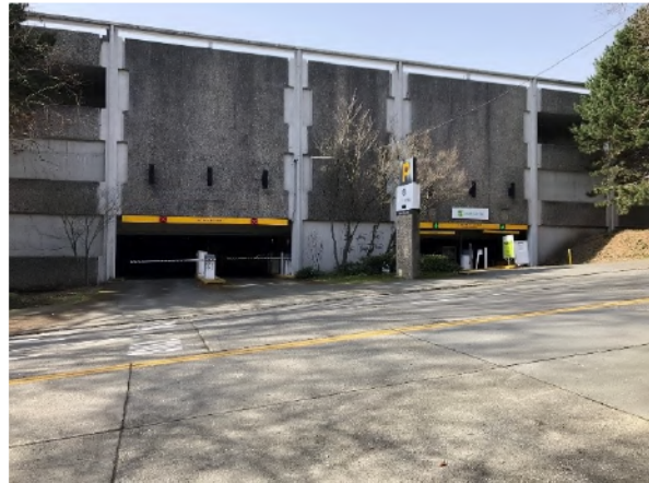
N - Mercer Street Garage – 4 th Avenue North Entry
