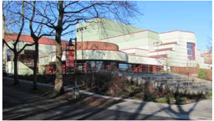
2013 image of the Seattle Repertory Theatre. Source: Artifacts Consulting, Inc.
