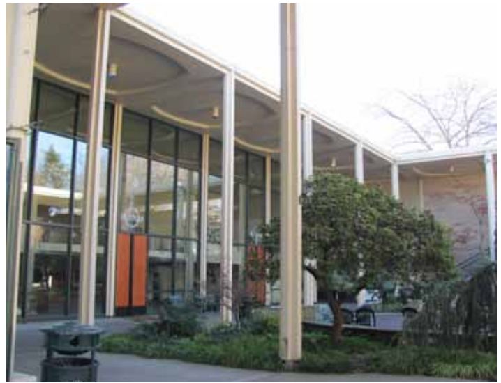
2013 view looking of the Playhouse courtyard. Source: Artifacts Consulting, Inc.
