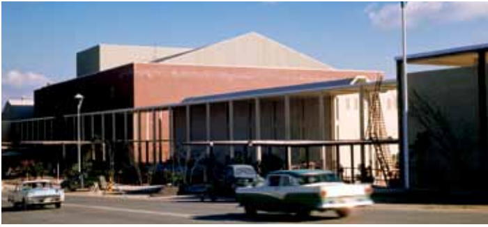
Historic view of the Exhibition Hall. Source: Mike and Carolyn Nore.
