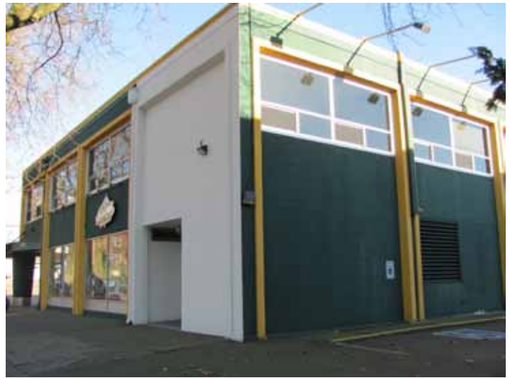
2013 view of the West Court Building. Source: Artifacts Consulting, Inc.
