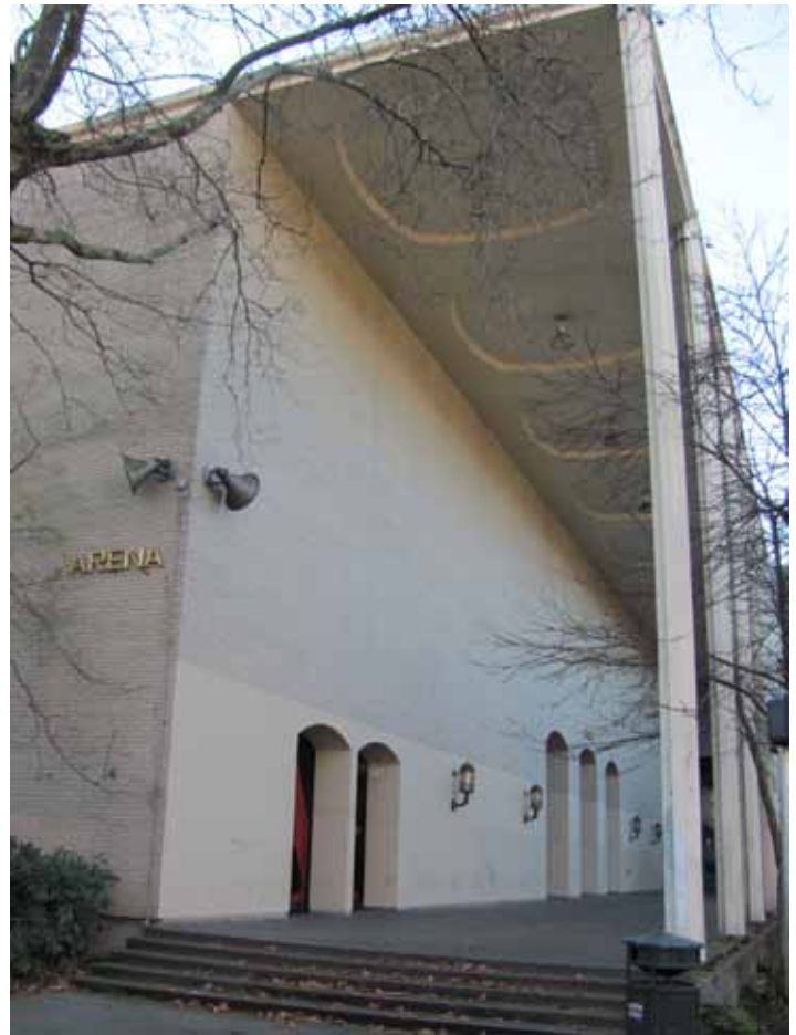
2013 image of the Mercer Arts Arena. Source: Artifacts Consulting, Inc.
